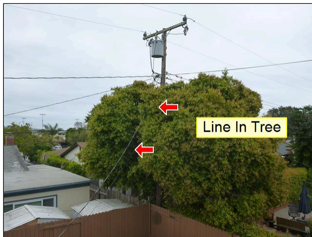
9.0 SERVICE / ENTRANCE LINE (See Picture(s))
